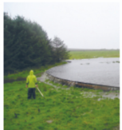
A pond that temporarily stores storm water before leaking it slowly back to the Belford Burn
